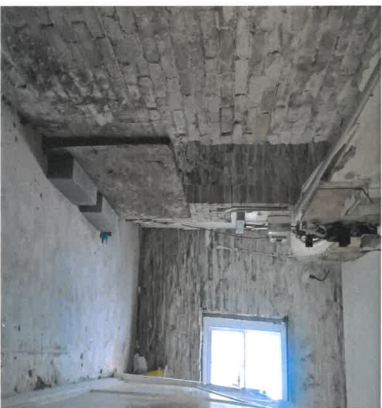
Station House Entrance After
